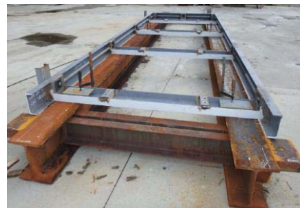
(b) Steel frame (top part)
