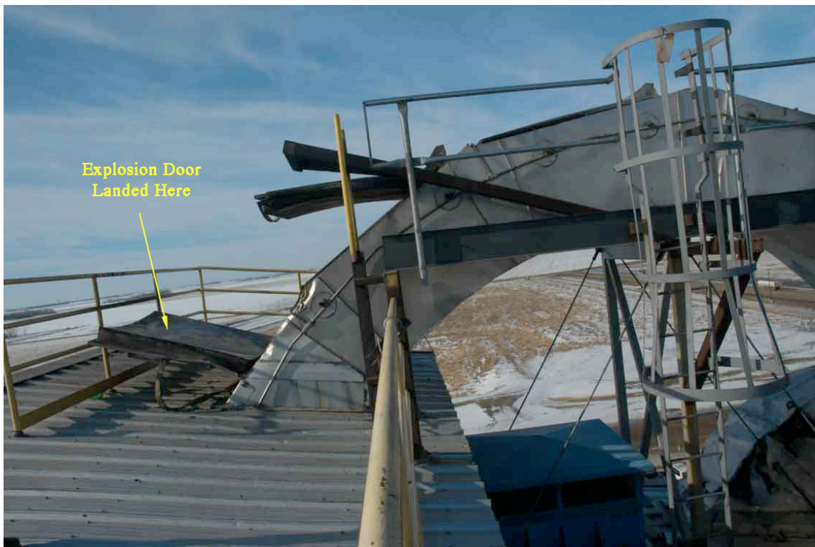
Figure 1: Explosion panel (door) from external ring duct that landed on the upper roof
