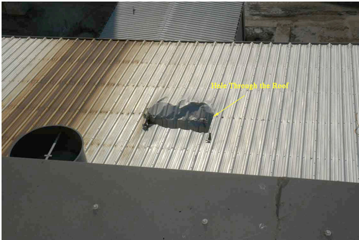
Figure 2: Explosion panel (door) that penetrated the roof
